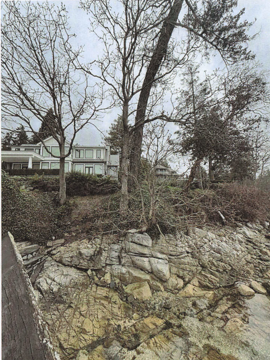
Plate #2. Typical view of existing conditions along the 15m marine DPA and the proposed retaining wall area. Works are proposed above the exposed bedrock
