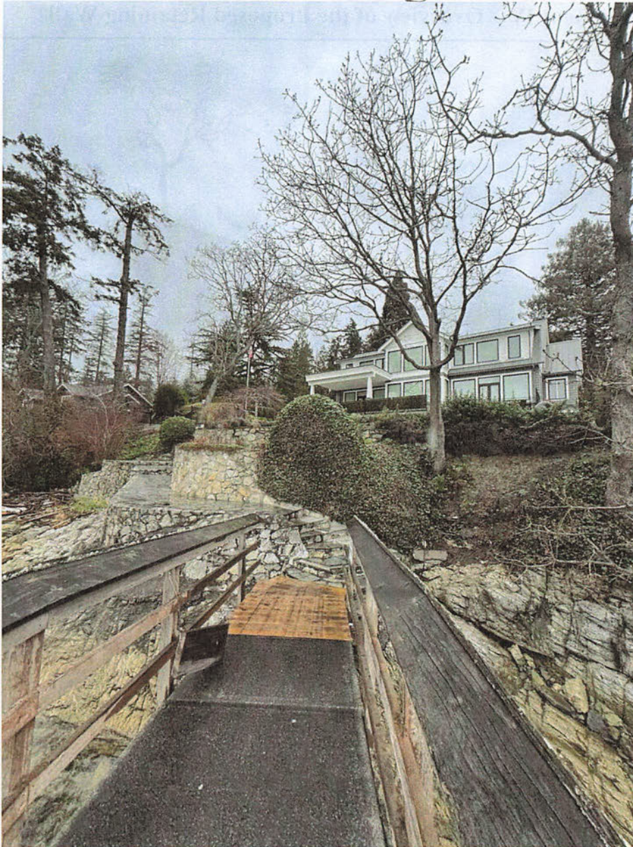
Plate #3. Typical view of existing conditions along the 15m marine DPA and the proposed retaining wall area. Works are proposed above the exposed bedrock
