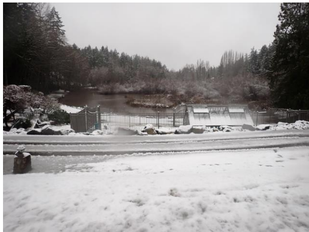
Photo 9: Pond @ 1:59 pm Recorded Water Level – Flooding around pond
