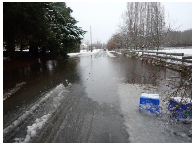
Photo 2: Munro Road @ 2:58 pm Recorded Water Level – 0.05 m over road
