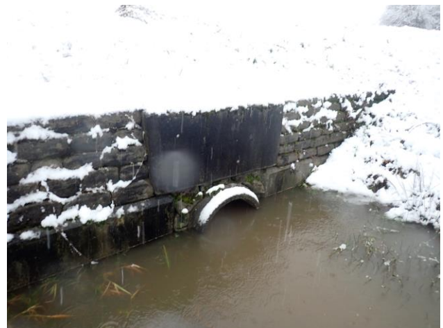
Photo 2: Outlet @ 12:35 pm Recorded Water Level – 0.53m (above invert)
