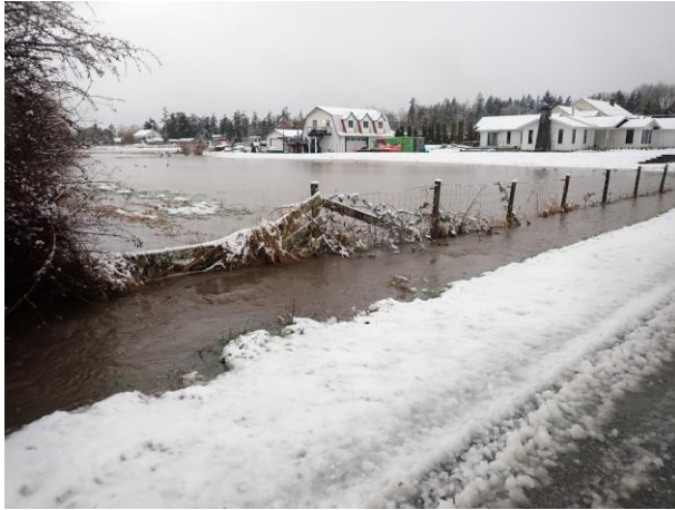
Photo 3: Outlet from Twin Culvert @ 1:30 pm Recorded Water Level – Fully submerged
