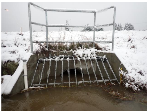
Photo 1: Inlet @ 12:30 pm Recorded Water Level – 0.66m (staff gauge)
