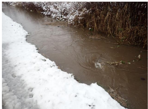
Photo 4: Inlet to Twin Culvert @ 1:30 pm Recorded Water Level – Fully submerged
