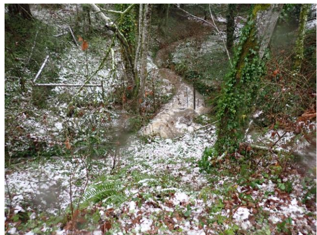
Photo 2: Culvert Outlet @ 2:05 pm Recorded Water Level – N/A
