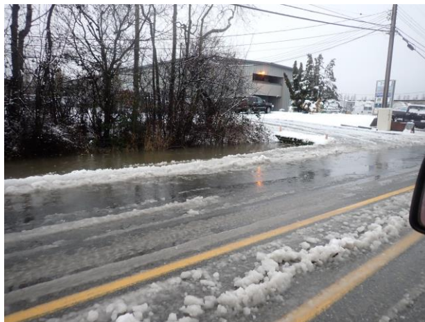
Photo 14: Culvert Inlet @ 2:34 pm Recorded Water Level – Submerged inlet
