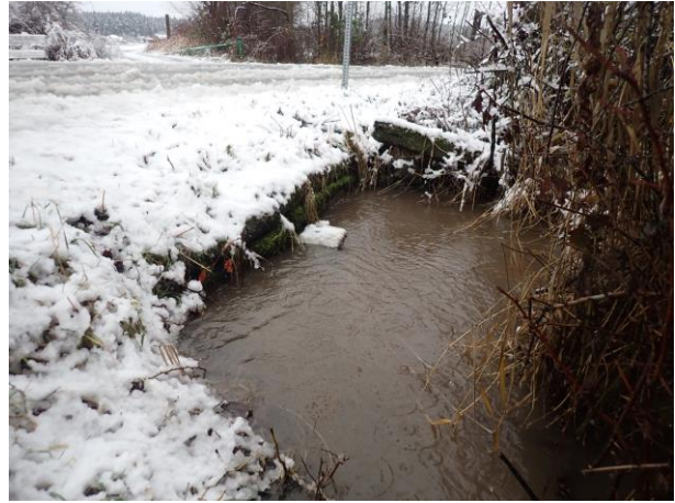
Photo 4: Inlet to Culvert @ 1:36 pm Recorded Water Level – Inlet fully submerged
