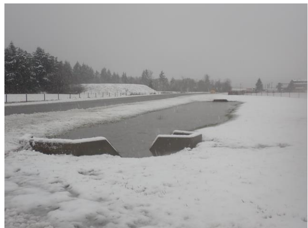
Photo 2: Culvert Inlet/Outlets @ 2:24 pm Recorded Water Level – Submerged
