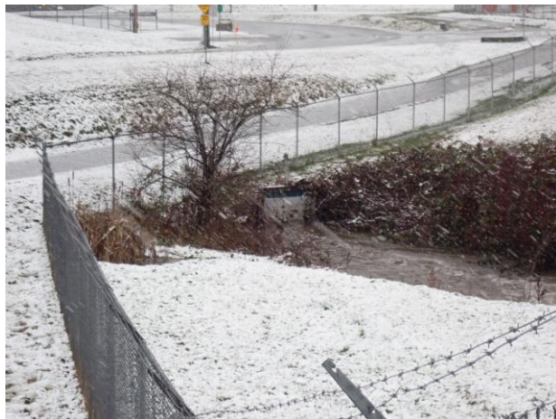
Photo 13: Culvert Inlets @ 2:28 pm Recorded Water Level – Submerged inlet
