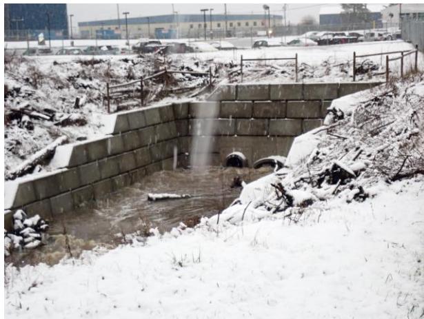
Photo 11: Culvert Outlets @ 2:14 pm Recorded Water Level – N/A
