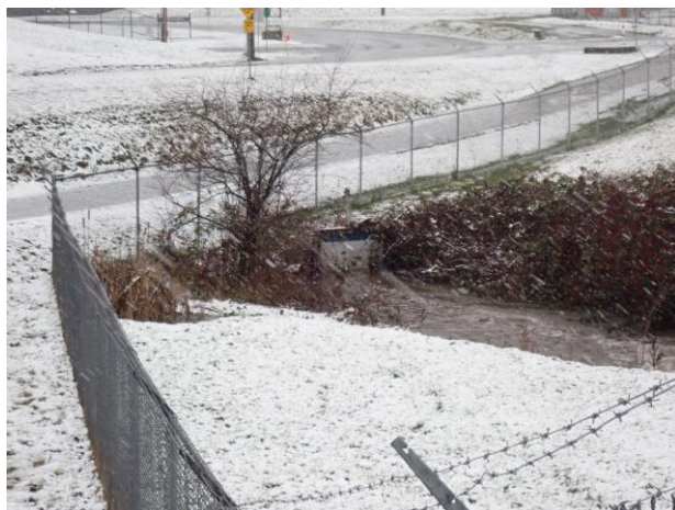
Photo 12: Culvert Inlets @ 2:21 pm Recorded Water Level – Submerged Inlet
