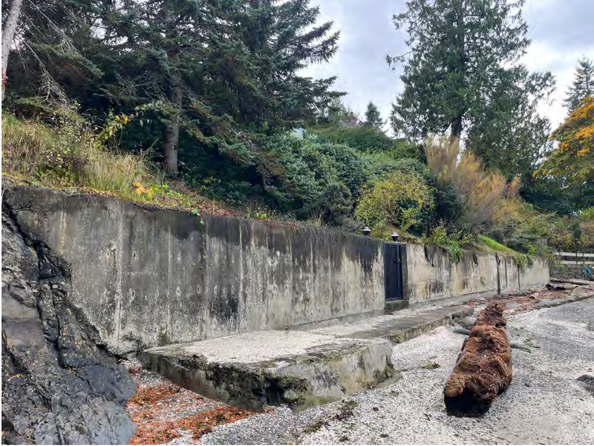
Figure 7. The adjacent property (906 Land's End Road) to the west of the subject property has a concrete retaining wall (~30 m in length), with a concrete toe extending into the upper edge of the intertidal zone. There is a gate (black structure) mid-way along the wall providing access to the shoreline. The next property to the west of 906 also has a mortared stone retaining wall (896 Land's End Road). These retaining walls were installed to prevent shoreline erosion of the riparian soils, lying behind the walls. There was no visible evidence of a stream discharging onto the shoreline on either 906 or 896 Land's End Road properties.
