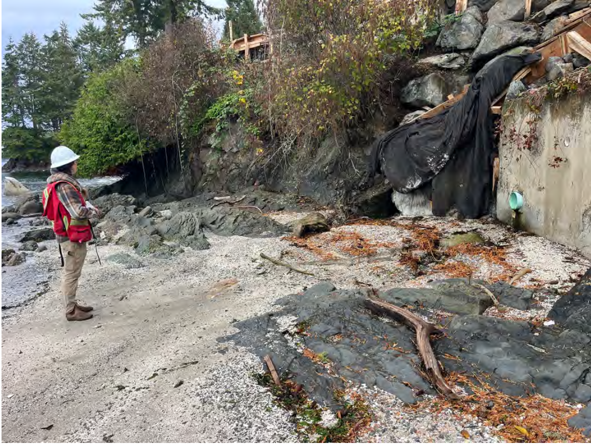
Figure 13. The western property boundary aligns with the concrete retaining wall on the adjacent property. Note the sandy beach sediments providing a thin, unstable cover on the bedrock shelves.
