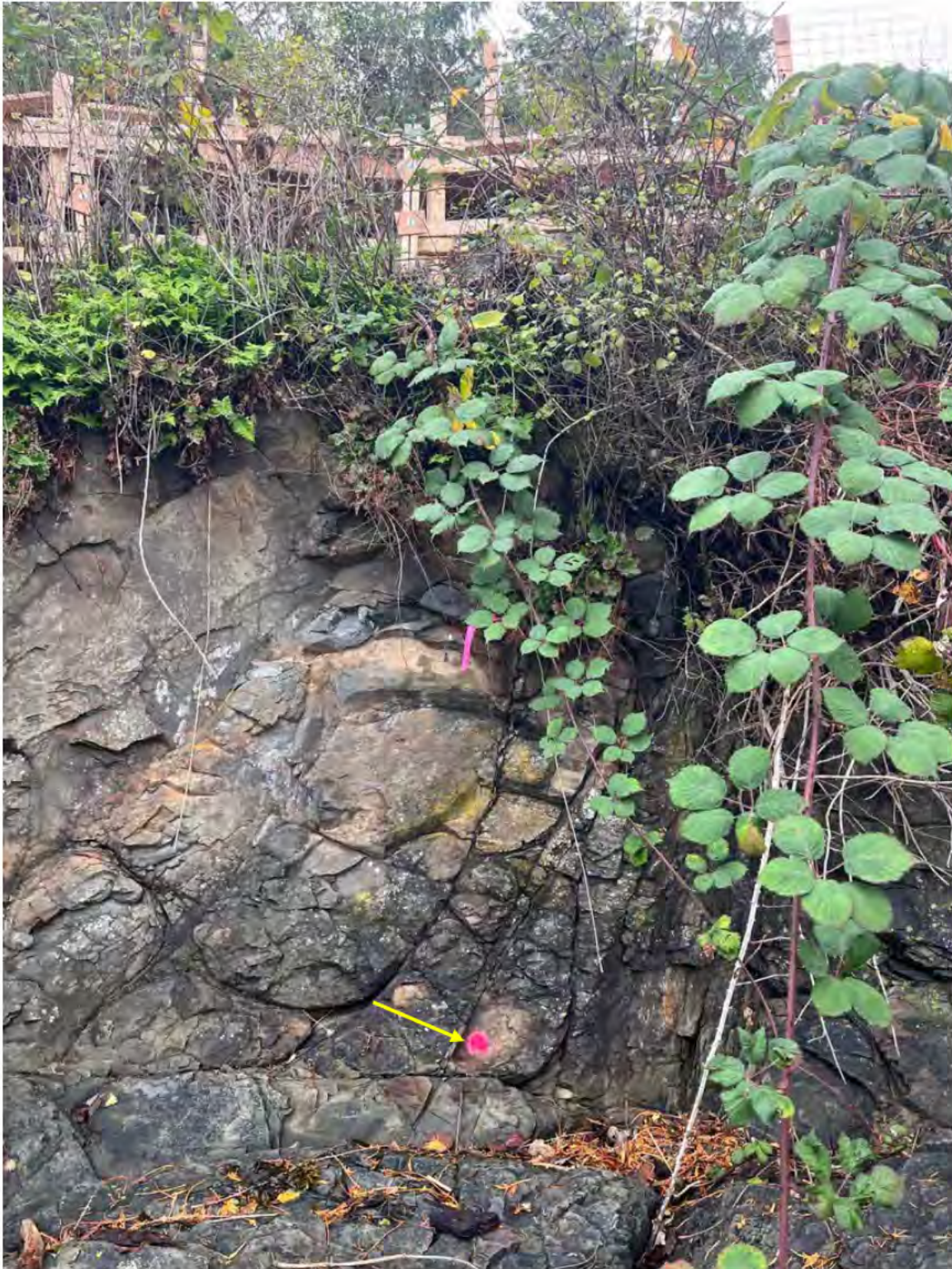
Figure 10. Typical bare bedrock slope with a thin plant covering. The wooden scaffolding will be removed at the end of the remedial works. The area seaward of the scaffolding will be planted with sword ferns. The yellow arrow indicates a red marker indicating the surveyed Present Natural Boundary (Figure 21).
