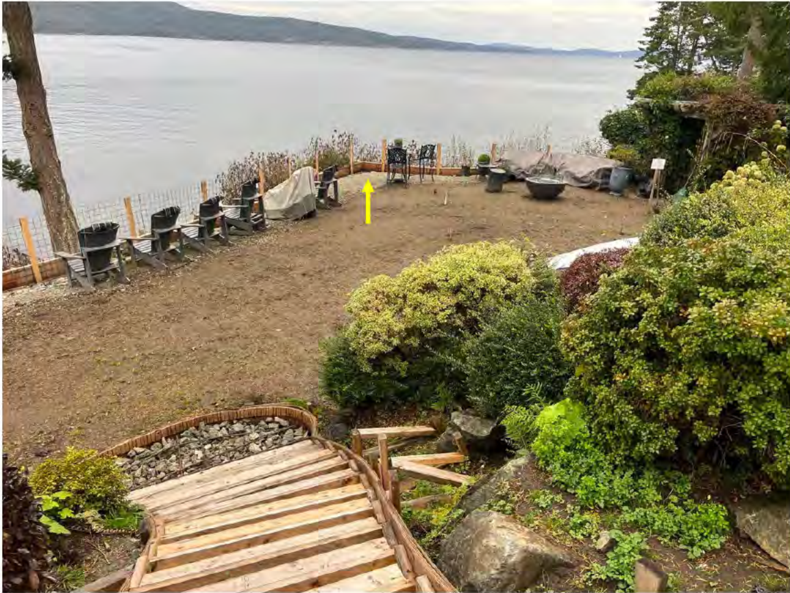
Figure 25. Preliminary landscaping works shown include leveling the lawn, the historical patio will be relocated away from the gate to the point of land (yellow arrow), the stairs linking the upper terrace to the lawn and stairs to the beach, the lawn edge on which the armoured glass fence panels will be installed (temporary mesh security fence), and the Douglas-fir tree.
