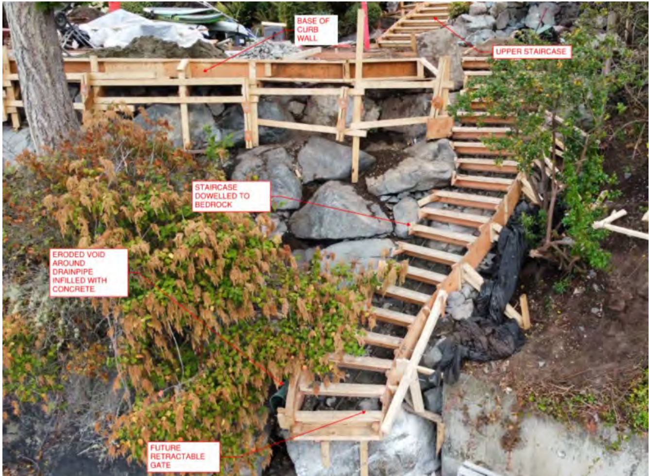
Plate 3: Looking South showing extents of staircase construction.
